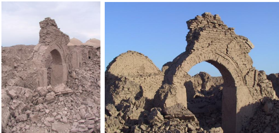
Figure 41 In-plane cracks, after the earthquake in 2003
