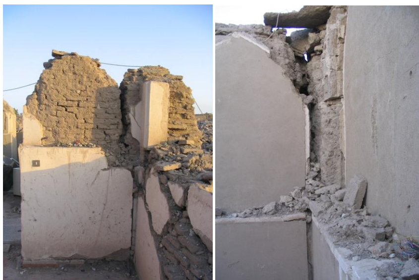
Figure 42 Cracks in the corner
