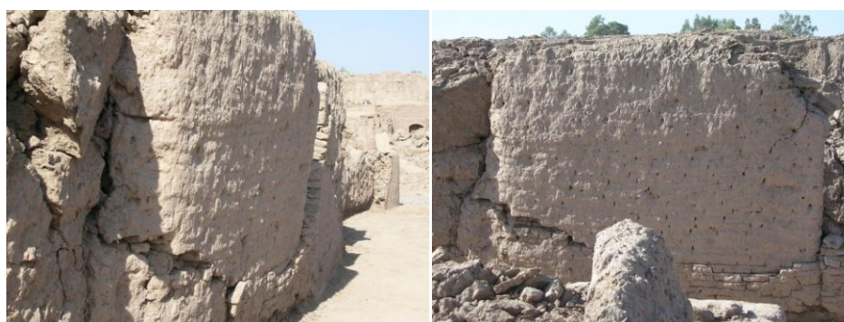
Figure 37 Horizontal and diagonal cracks after Earthquake, 2003.
