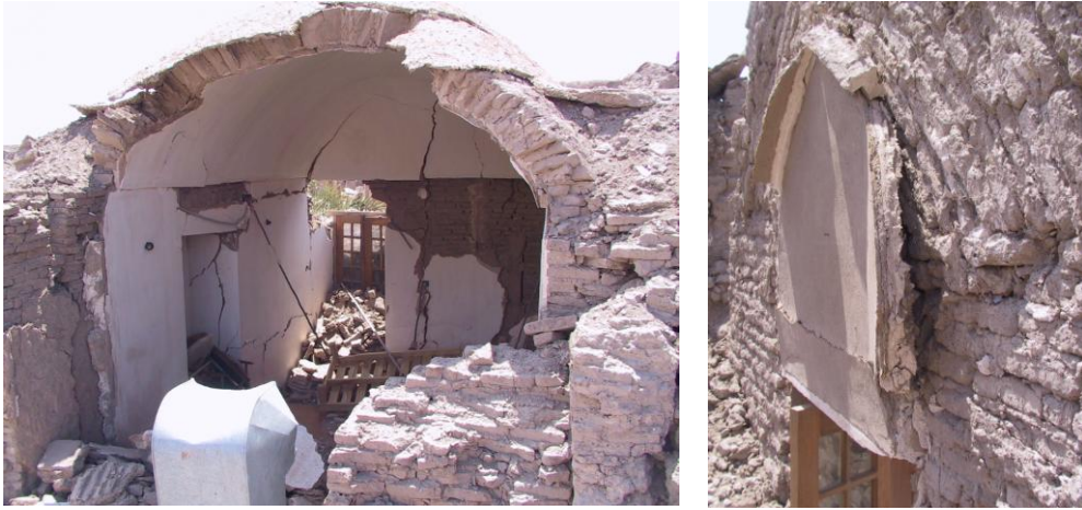
Figure 43 Cracks and crash at openings
