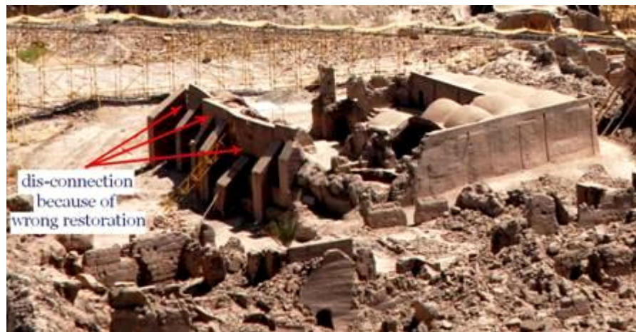
Figure 50 Collapse because of neglect of the engineering calculation for the buttress, [53]
