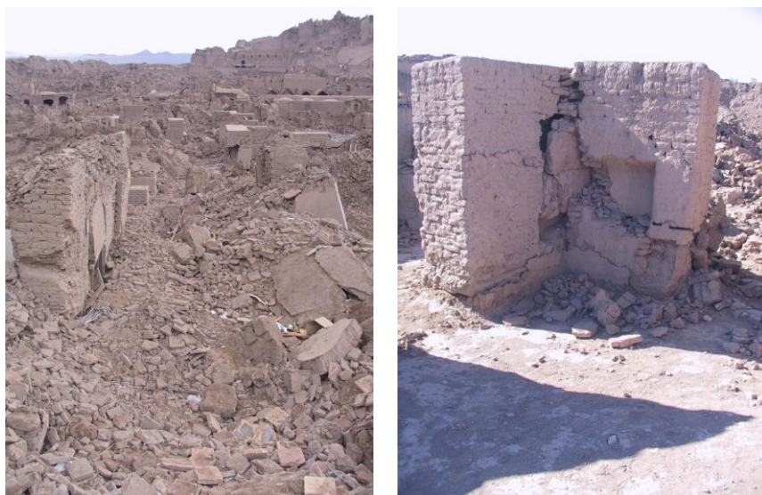
Figure 38 Cracks, crashing and collapse after Bam Earthquake, 2003
