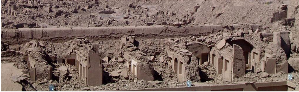
Figure 40 Out of plane walls, remain following the earthquake in 2003.
