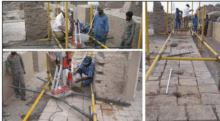
Figure 73 Drilling procedures for inserting vertical Siess elements in the main walls in Pyambar Mosque, [47].
