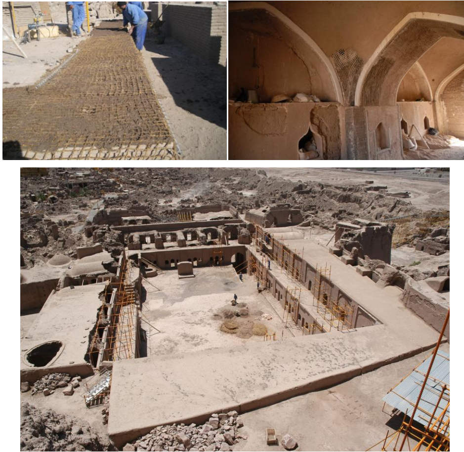
Figure 83 Applying meshes in Small Storage, Stable, and lightening in Barracks
