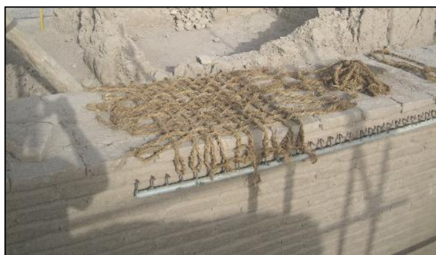
Figure 74 Horizontal Siess were inserted among the layers [47].
